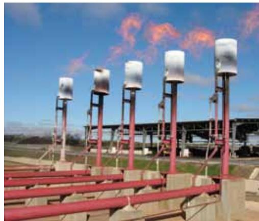
SAWS burned off the methane produced as a by-product of the anaerobic digestion process from biosolids. Now, Ameresco treats the gas and transfers it into a commercial gas pipeline as a green energy source.
